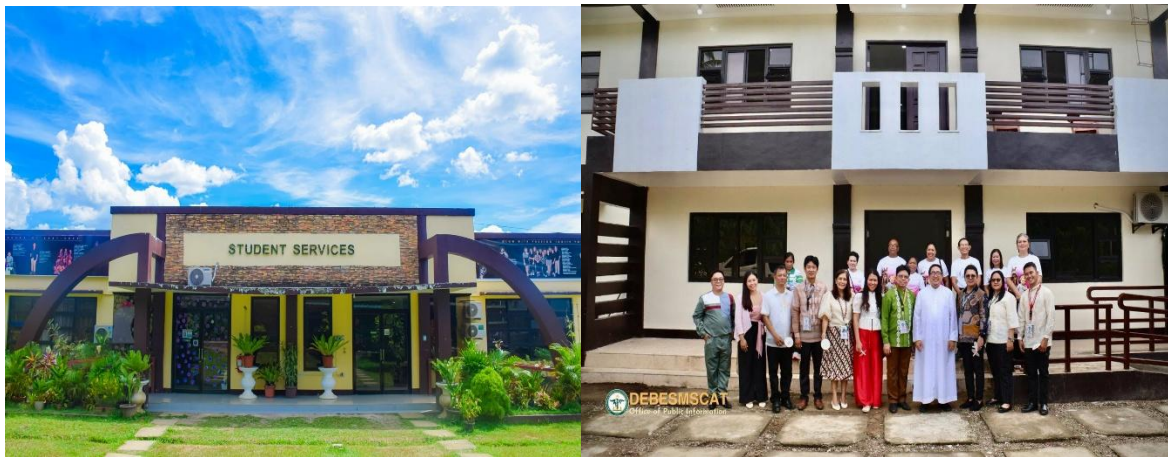
Figure 45. One-Stop Shop OSAS Building
